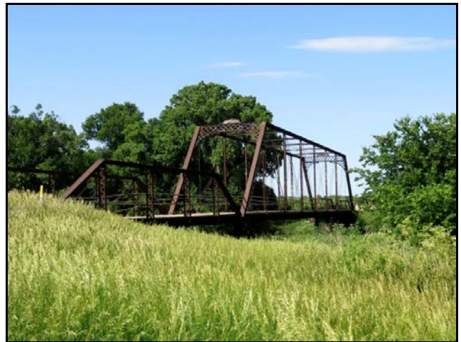
The old river bridge is currently closed to vehicular traffic.
