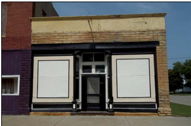
The Biggs building, the oldest on Main Street, just received fresh paint this summer. How many times has it been painted since new in 1880?
