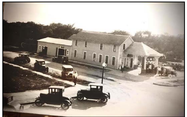
Glasco: looking southwest at Main and Railroad
